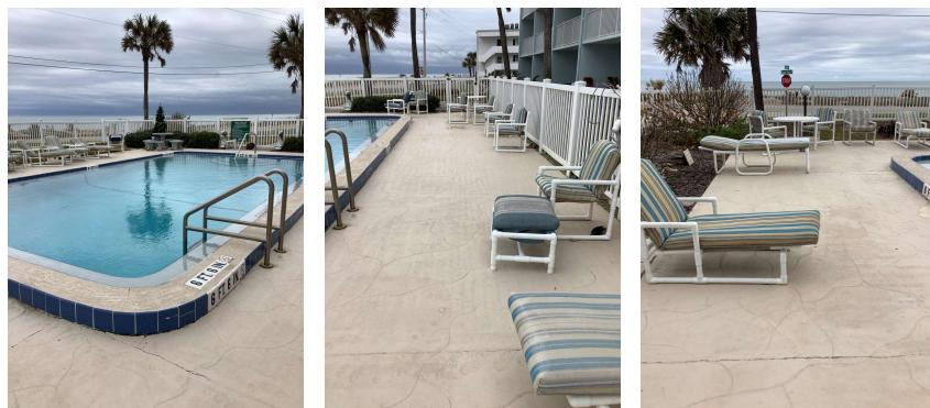
This category refers to costs associated with the replacement and repair/ resealing of concrete/ paver pool decking areas. Barring unforeseen damage, and assuming proper and routine maintenance, a minimum useful life of approximately 25 years can be expected. The current replacement cost estimate is based on industry standards, national cost estimating indexes, and our experience with this type of component.
