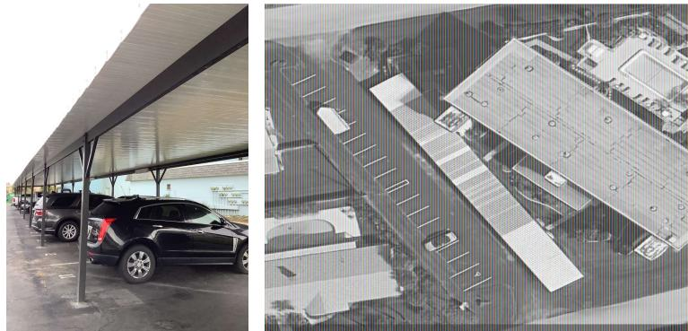
Metal roofing approximately 3,368 sq ft. Data gathered from within the local market suggests a probable life cycle in the 35-40-year range for a professionally designed, installed, and maintained roof including gutters. The current cost estimate includes removal and disposal of the existing roofing,
