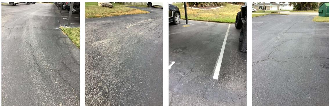
This category refers to costs associated with the milling, recoating, and striping of asphalt parking areas. Barring unforeseen damage, and assuming proper and routine maintenance, a minimum useful life of approximately 15 years can be expected. The current replacement cost estimate is based on industry standards, national cost estimating indexes, and our experience with this type of component.
