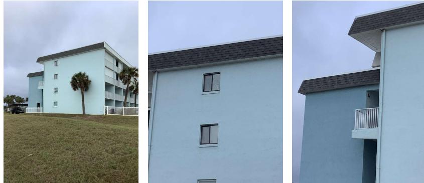
Mansard shingle roofing approximately 1281 sq ft. Data gathered from within the local market suggests a probable life cycle in the 20-25-year range for a professionally designed, installed and maintained roof. The current cost estimate includes removal and disposal of the existing roofing, typical minor repairs to the underlying roof structures, flashing, etc. and installation of like roofing.
