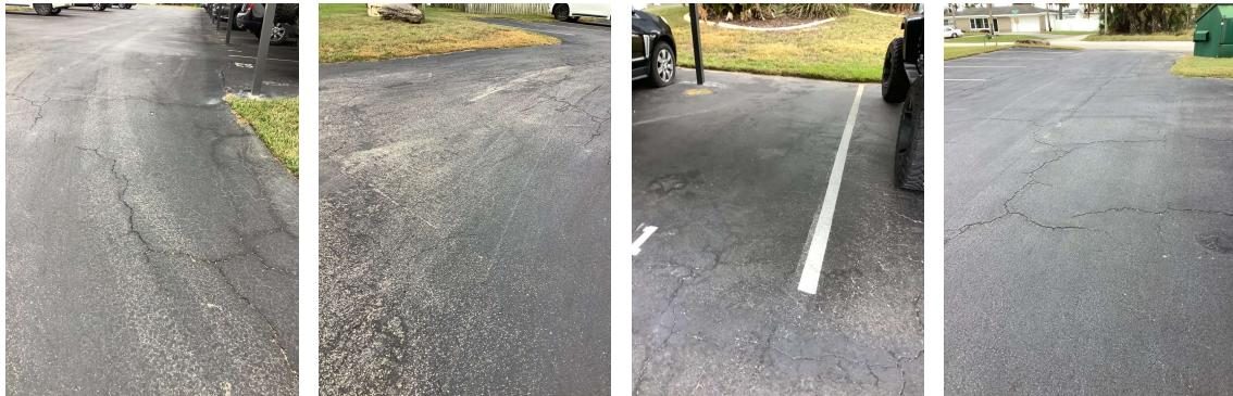
This category refers to costs associated with the seal coating of asphalt parking areas. Barring unforeseen damage, and assuming proper and routine maintenance, a minimum useful life of approximately 5 years can be expected. The current replacement cost estimate is based on industry standards, national cost estimating indexes, and our experience with this type of component.
